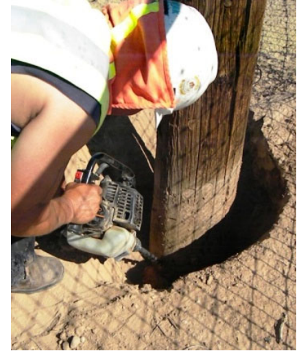
2-Drilling and digging below GL
