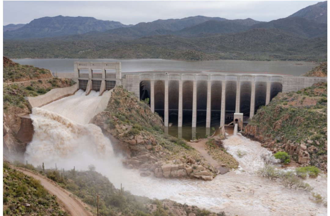
Barlett Dam water release
