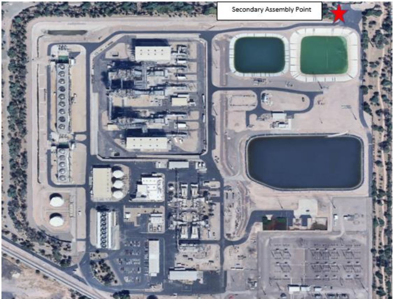
Santan Generating Station Secondary Emergency Evacuation Assembly Area
