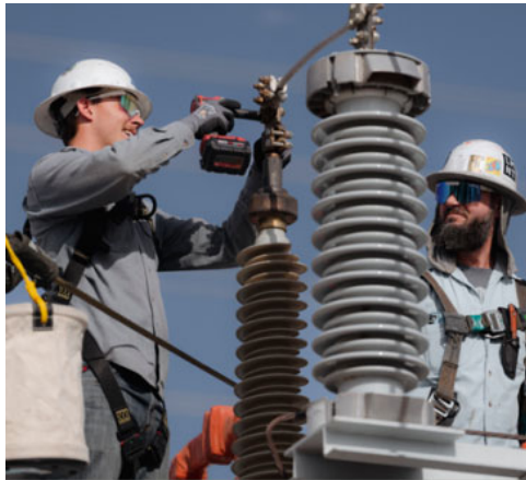
LJ Muth (left), Pre-Apprentice Substation Electrician, and Joey Murawa, Substation Electrician, remove conductors from bushings on a 69 kV transformer.
