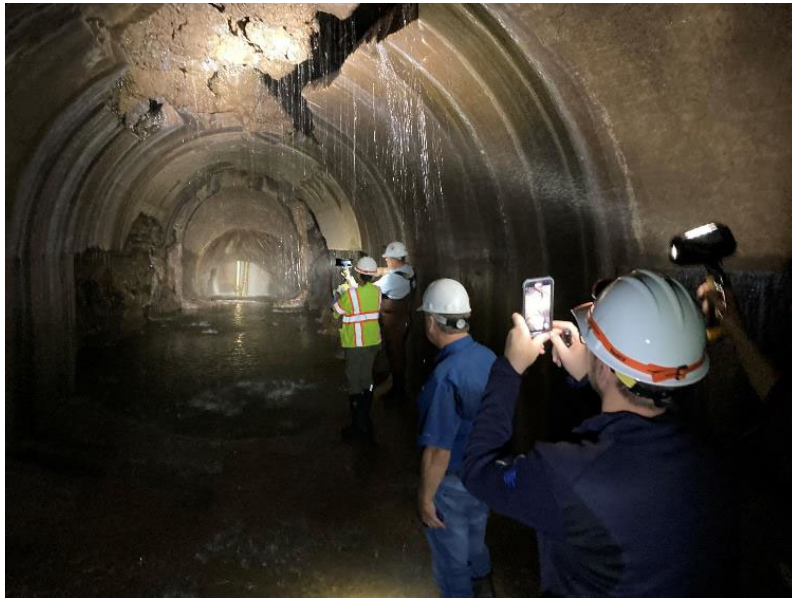
BOR and SRP staff inside ROW tunnel on 7/31/2023
