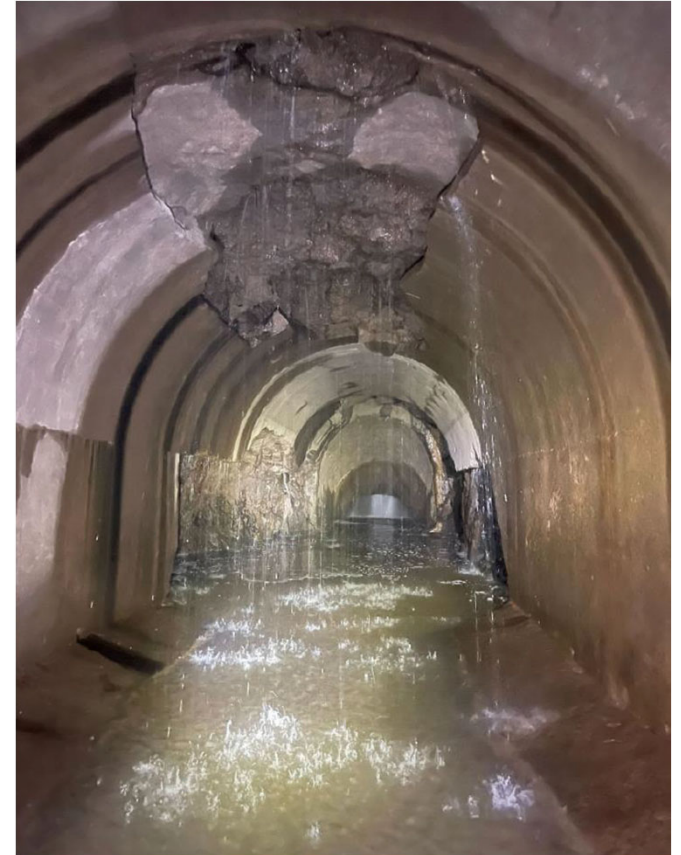
Looking upstream, past bend, just downstream of drum valve
