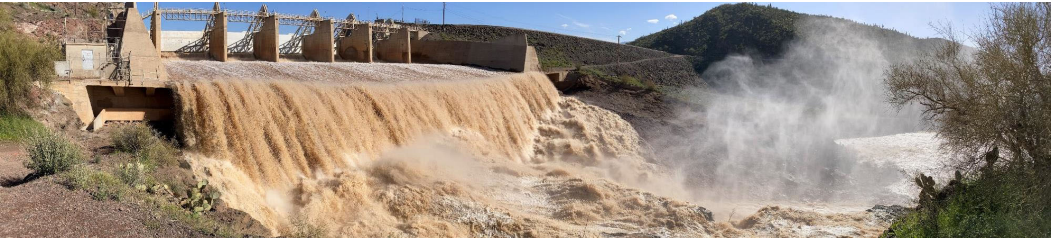
Water releases at Horseshoe Dam during winter runoff, March 2023
